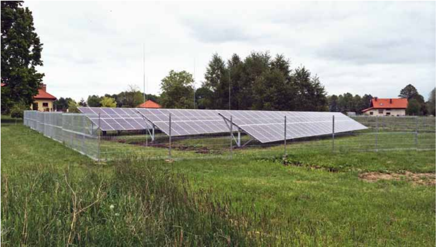
PV arrays up to 40 kW, such as this array in Bojszow, are largely free from regulations, empowering the prosumer.
